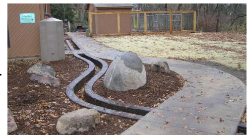
The rain canal takes water from a rain barrel to the rain garden.
