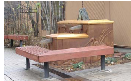
A rain chain directs roof runoff in the rain planter.
