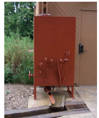
The rain canal takes water from a rain barrel to the rain garden.
