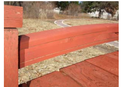
Bridge lets Water Flow Below
